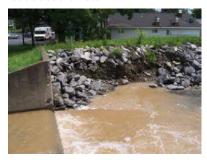
Deflection dikes, plastic sheeting, snow fencing and other material may be used to arrest scour and erosion. Lavers of protective materials (such as plastic sheets) should overlap in a manner similar to the placement of roofing shingles, with the edge of the upstream
