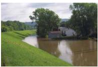
The discharge from portable pumps is strong and can lead to erosion of levee material. Check for possible scour damage as a result of pump discharge. Communicate observations to the patrol leader/coordinator.
