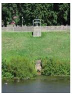
gate should be lowered (closed). This is done from the hoist at the top of the structure. To permit drainage of ponding areas, sluice gates lowered during a high-water event must be raised after river levels subside. Flap gates should then be checked for proper operation.
