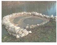
to stop the water flow as other sand boils may occur outside the sandbag ring. Discharge from the sandbag ring should be diverted away from the levee or floodwall to the nearest drainage structure or ditch when practical.
