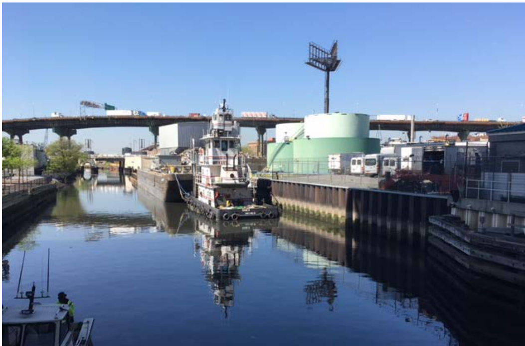
The Gowanus Expressway/Hamilton Avenue Bridge crossing over the Gowanus Canal. Photo courtesy of R. DelVecchio.
