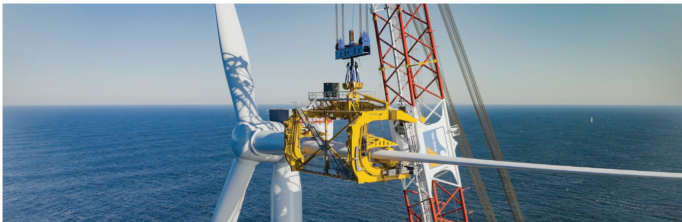
An offshore wind turbine under construction.
