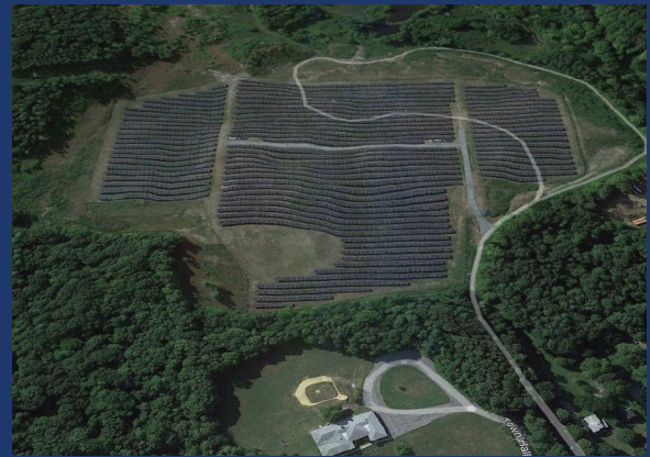
An aerial view of the Irish Hills solar array.
