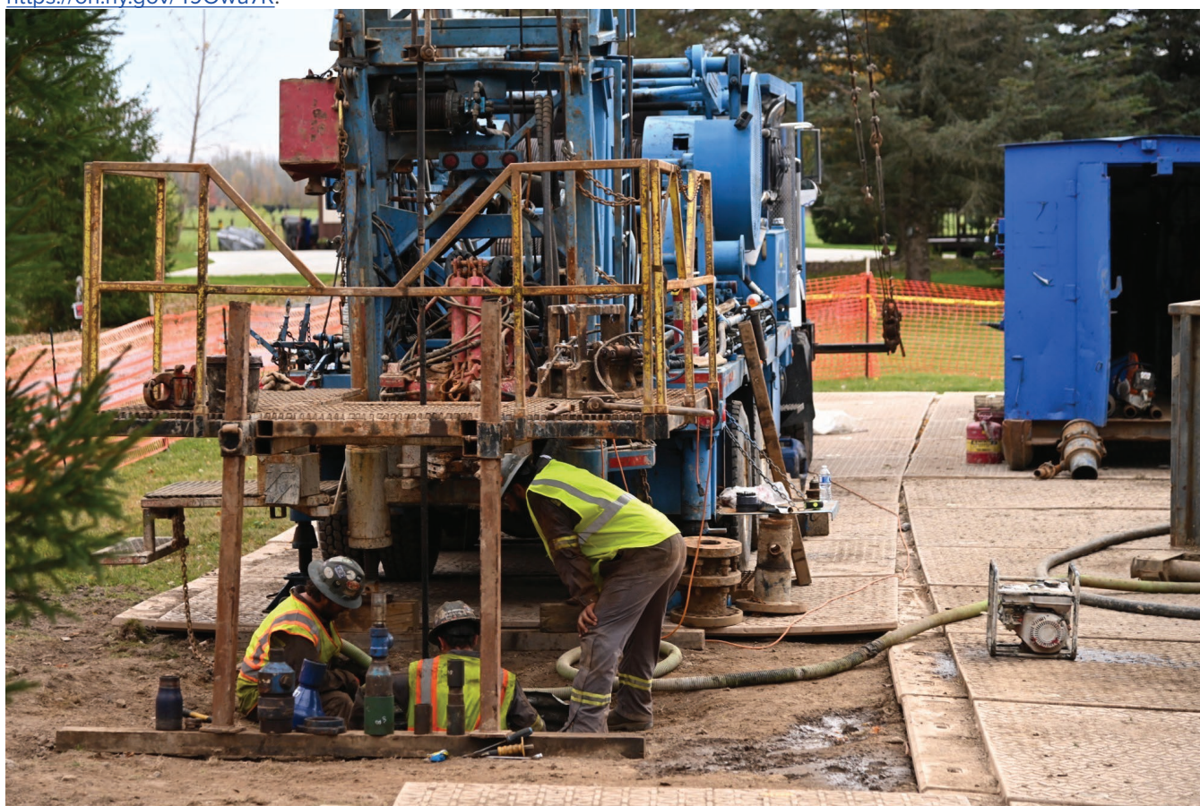
Workers plugging an orphan well.
