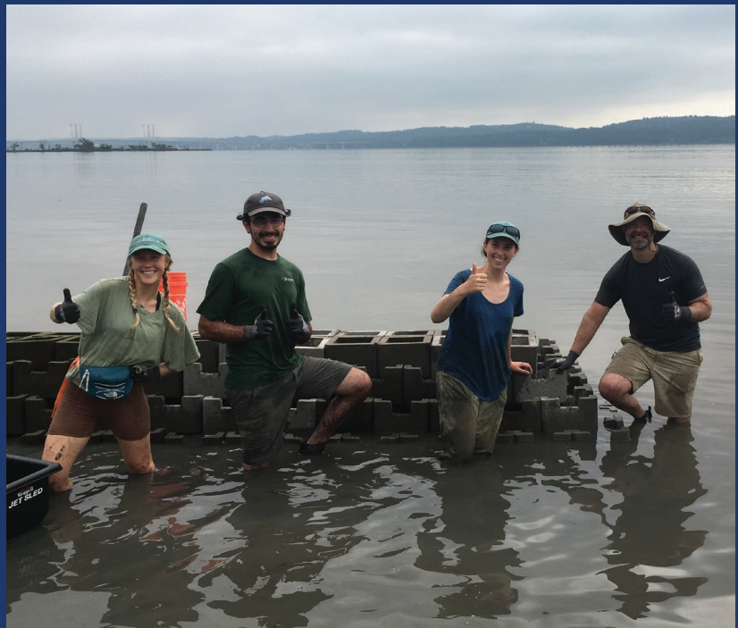
Staff and volunteers installed more than 8,000 oyster castles as part of the Piermont Marsh stabilization project.
