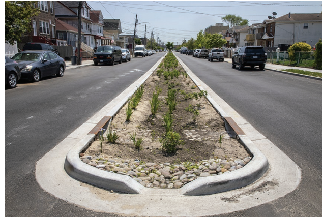
Before (above) and after green infrastructure project in Queens.
