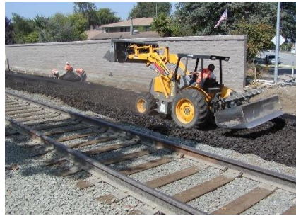
Figure 9: TDA placement alongside tracks
