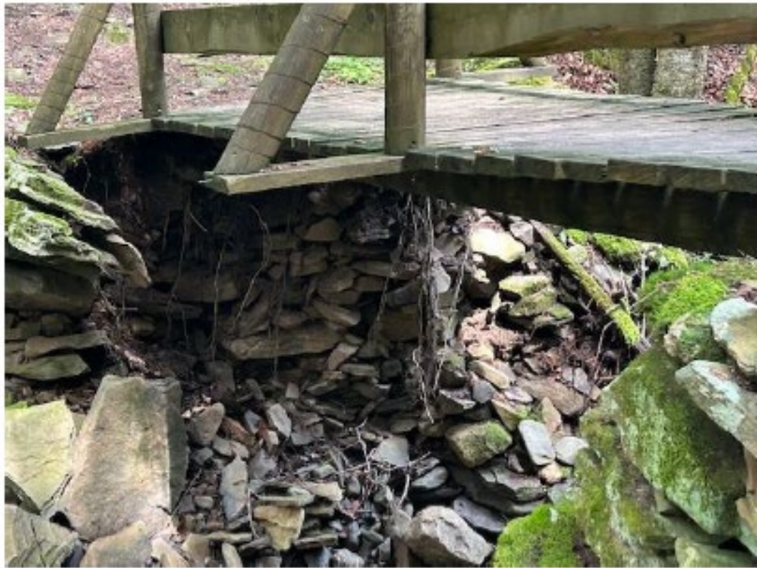
Figure 2: Collapsed Abutment
