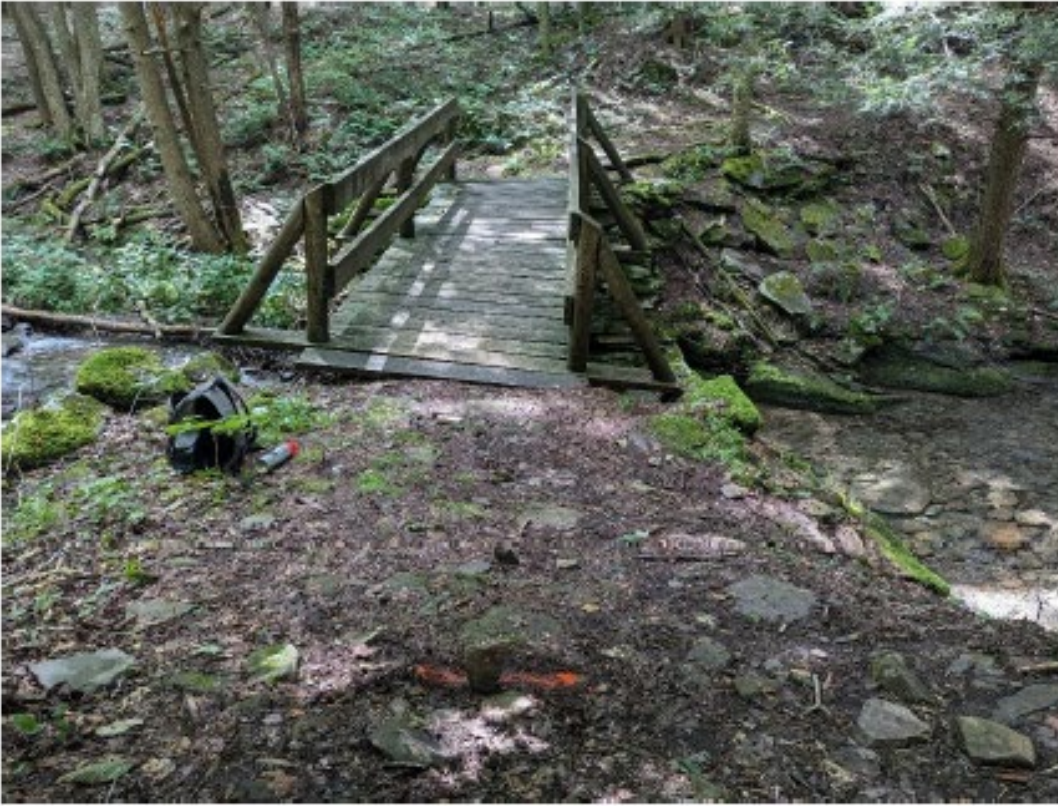
Figure 3: Proposed new abutment in orange paint
