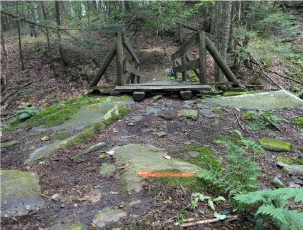
Figure 4: Proposed abutment in orange paint
