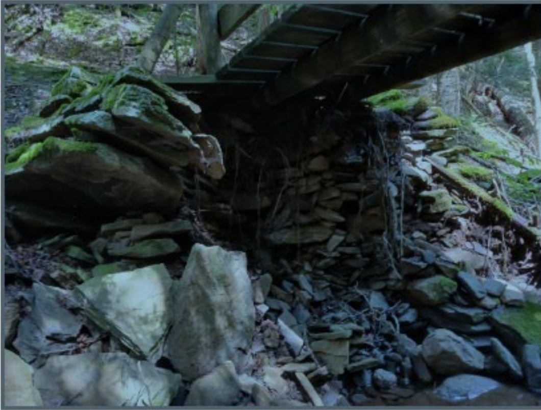
Figure 1: Collapsed Abutment
