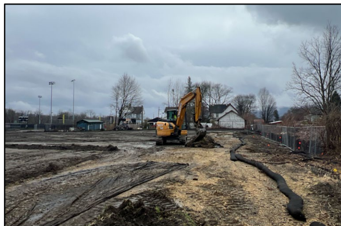
Figure 2: April 2024 – Restoration Activities in NAF
