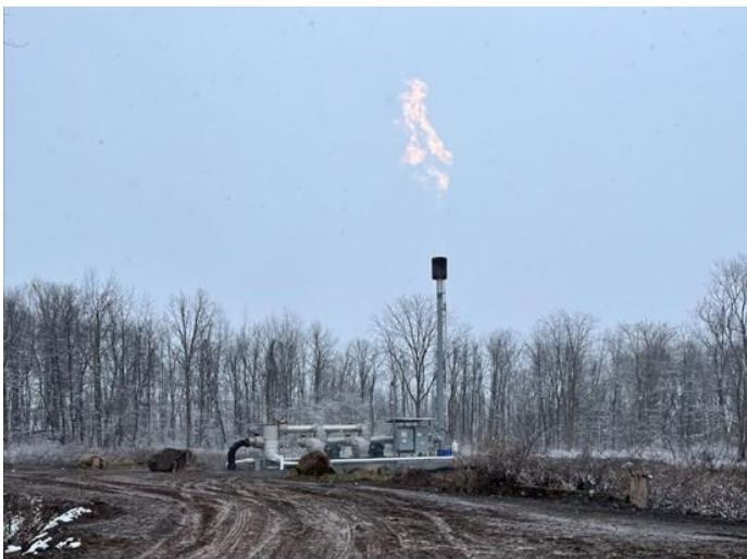
Utility flare relocation and replacement.
