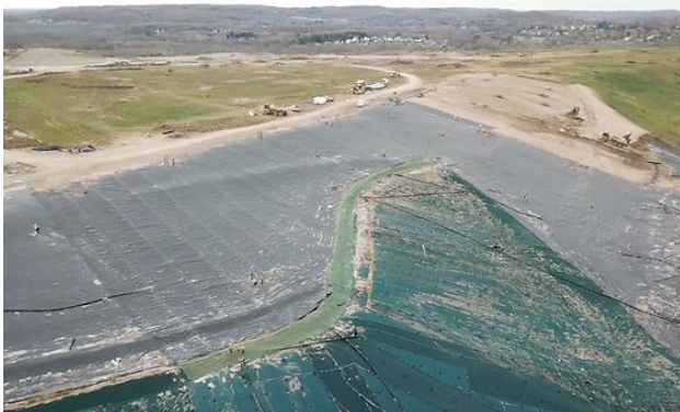
Geomembrane cover installation on the north side slope, Fall 2024.
