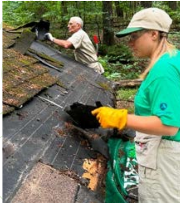
Steward Anna removing the old roof shingles
