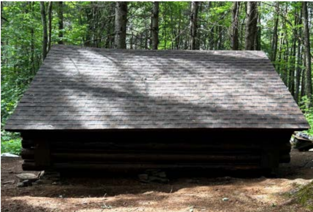
The new and improved roof on the Elm Ridge lean-to
