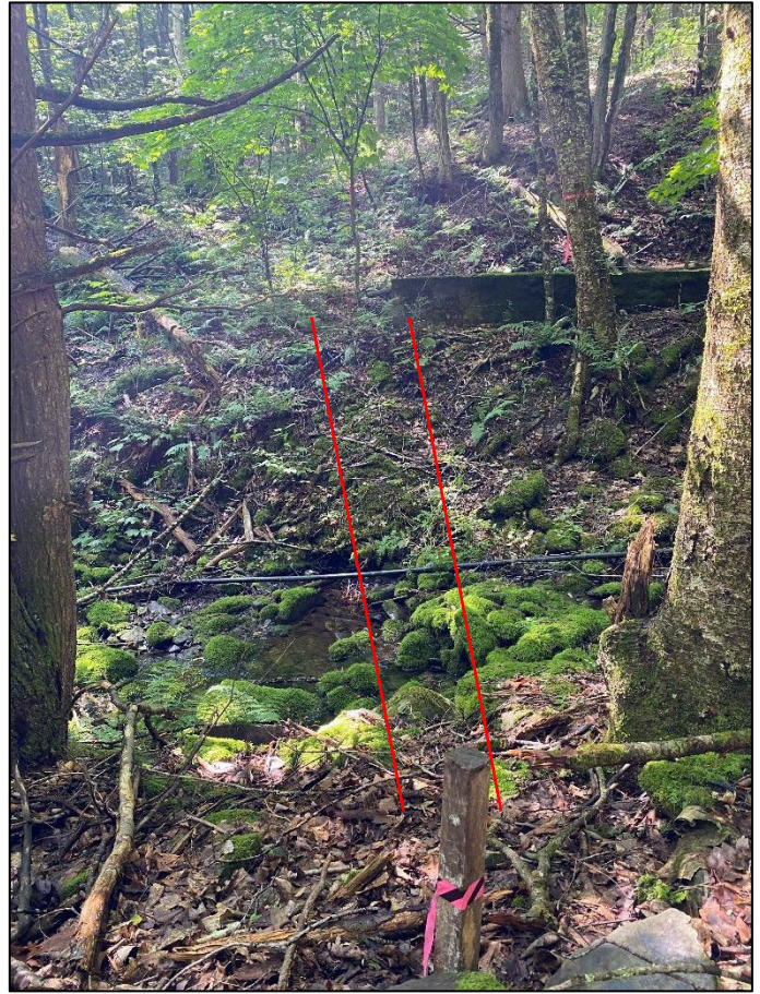
Approximate location of the 32' span 4' wide bridge. Note the cistern on the right-hand side.
