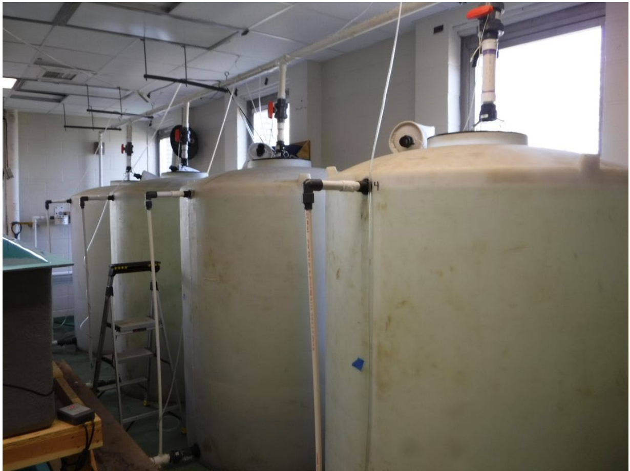
Figure 2-3: Seawater holding tanks for the Mesocosm experiments
