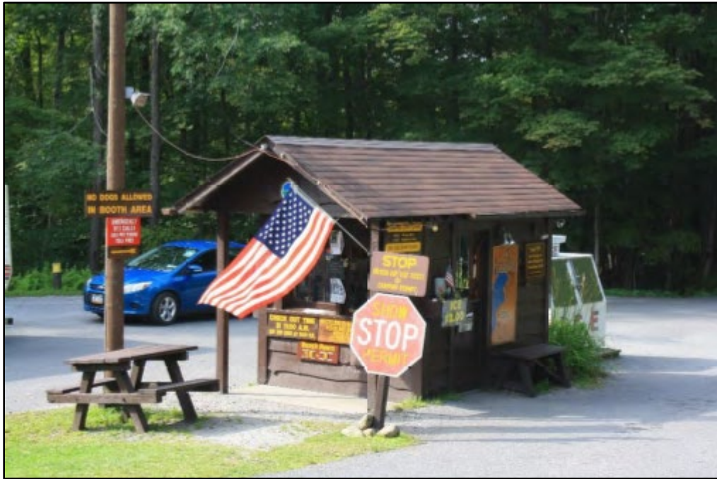
Figure 2 – Existing Ticket Booth
