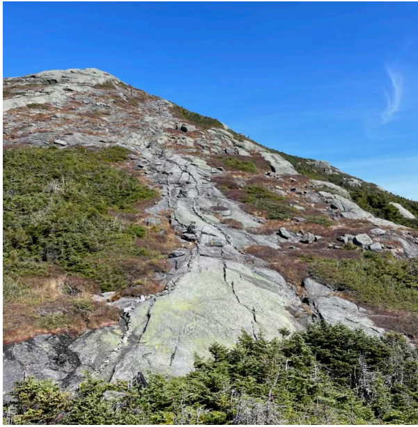
Completed scree wall on backside of Marcy
