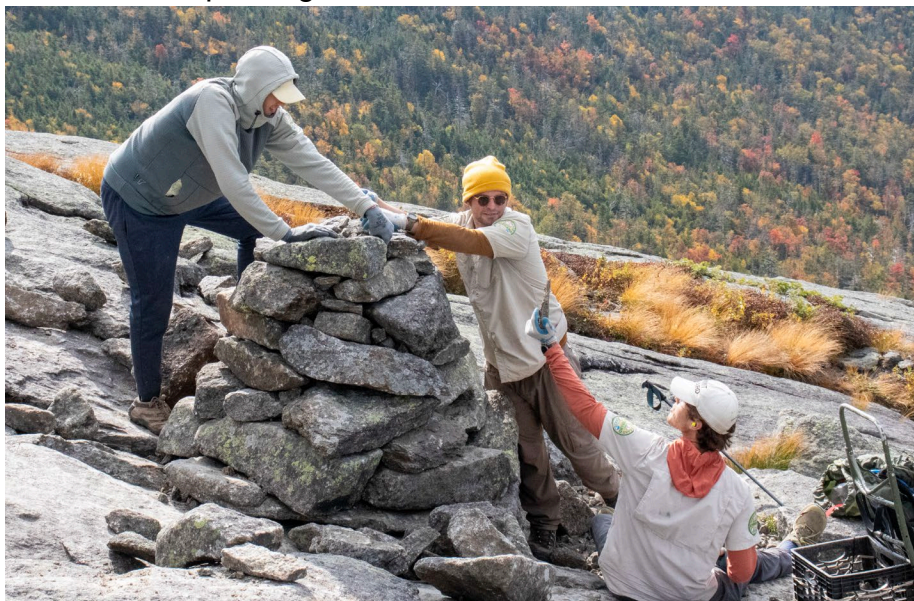
Ryan, Eli, and Chris filling their cairn with crush. Crushed rocks help stabilize the cairn and make it a solid and dense marker.
